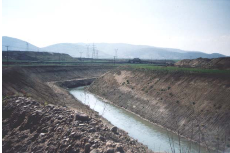
Fig. 22 Bed adjustments of Soulou torrent near LCWM
